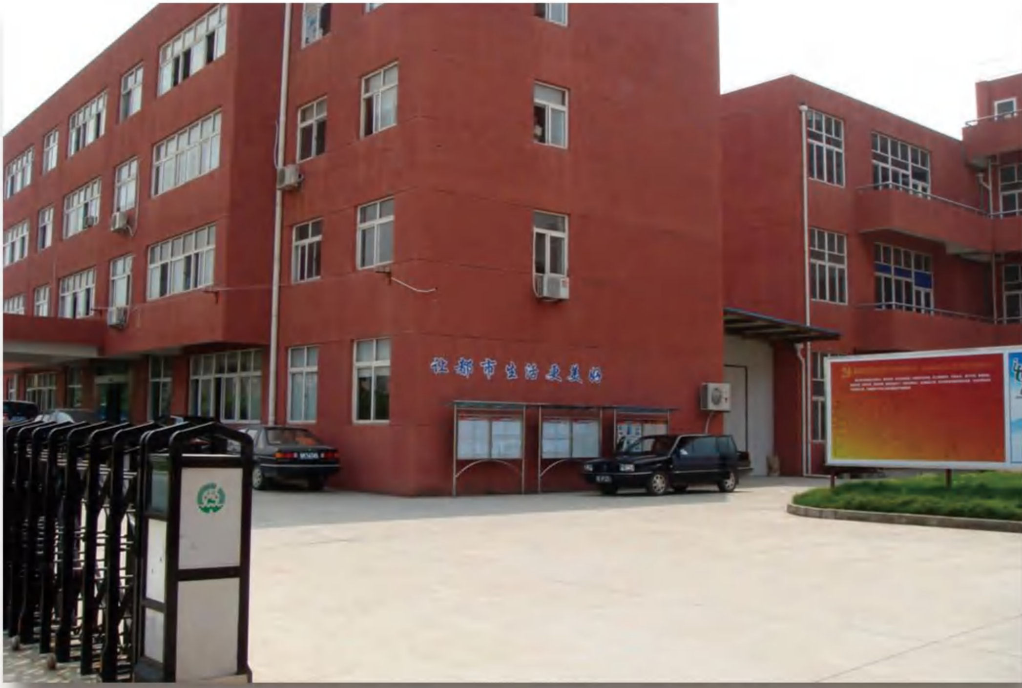
厂房大楼 Factory building
